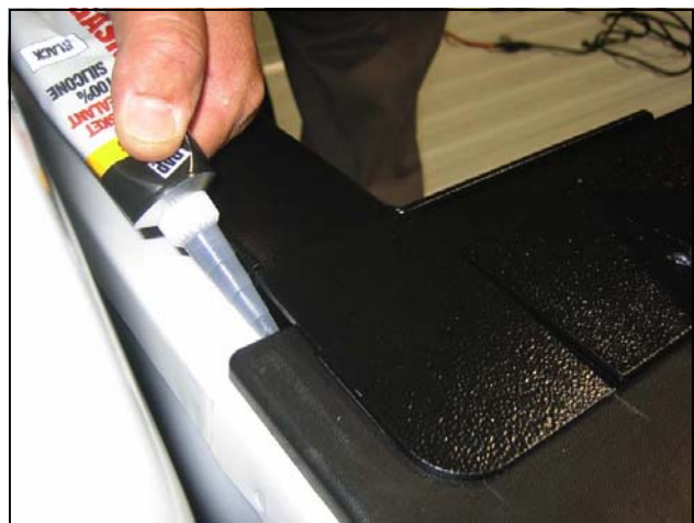
At each front corner, caulk the gaps shut with the RTV supplied in the installation kit.
